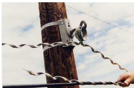
4. Place the paint mark of the reinforcing rod on top of the cable vertically to the pigtail. Wind up the reinforcing rod around the cable on total length.
