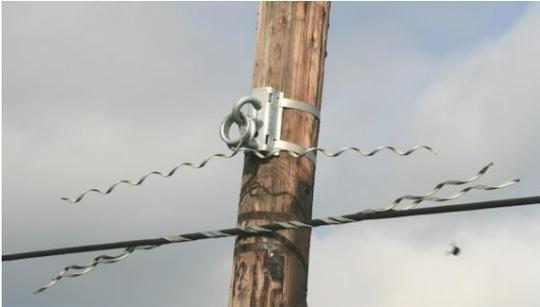
5. Wind up simultaneously the two branches for two or three pitches. Complete the assembly of the two branches around the cable on the total length. Take care to avoid to damage the cable outer jacket with the wire tips (see the note below).
