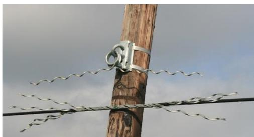
3.5 At both ends complete simultaneously the winding of wire sets.
