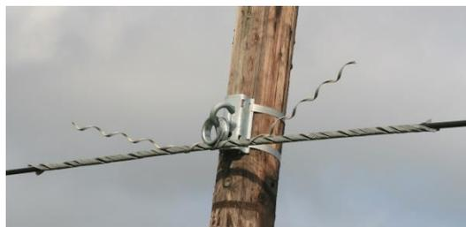
4.1 Position the cable with protecting rods between the two legs.
