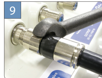
Tighten connector to recommended torque.
