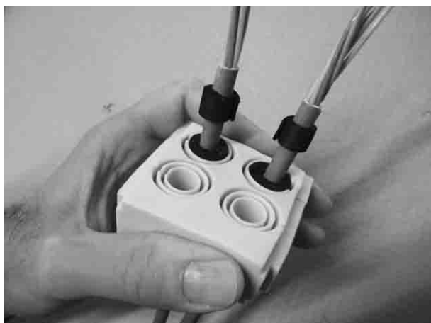
Use the foam to fill the gap between the jacket of the cable and the port of the block. Install the cable into the block.
