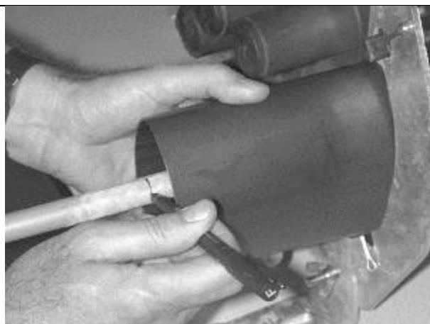
Remove the packing bag out of the seal, push the seal upwards to the base and mark the cable flush with the seal. Make sure the seal butts up against the base.
