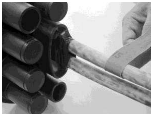
Clean and abrade the cable
